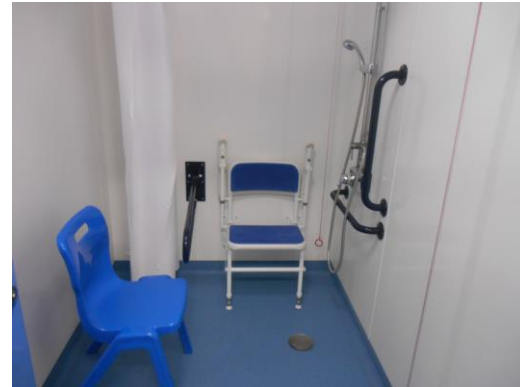
Picture 5: Ward 2 South, refurbished, well-presented shower room
